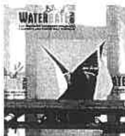
On arrival of doors and windows, cut the WATERGATE PLUS at each opening on a 45° angle away from each corner. Pull the WATERGATE PLUS flaps inside and fasten to inside of frame.
