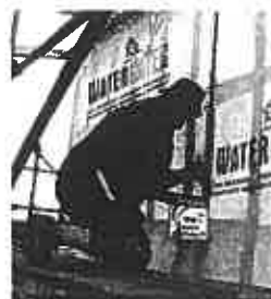
Application of Thermakraft Stud Strap for cavity construction where studs spaced > 450mm.
