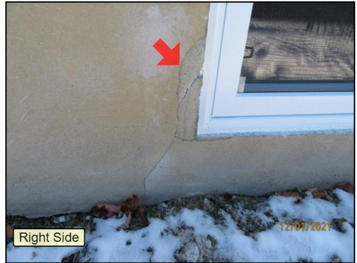
34. Grouting damaged or missing
