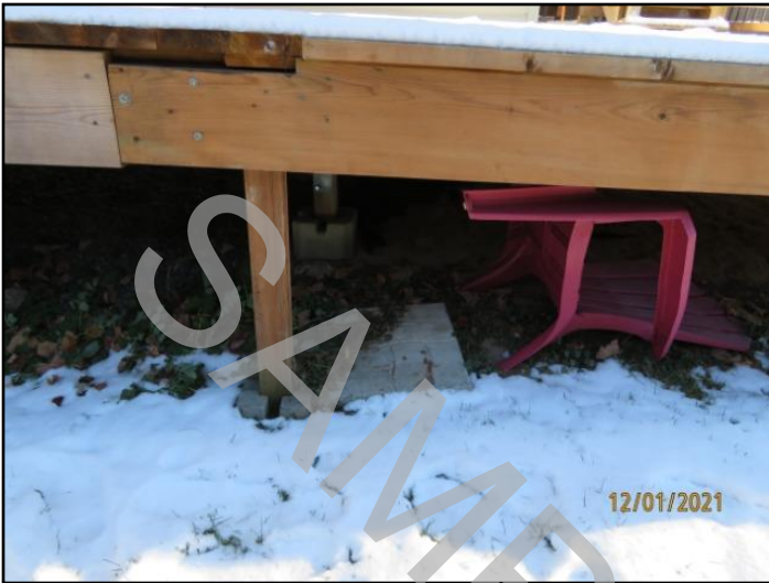
12. Poorly secured at top & bottom:At the...
