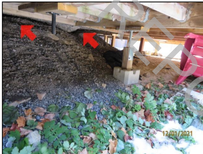
14. Wood/soil contact
