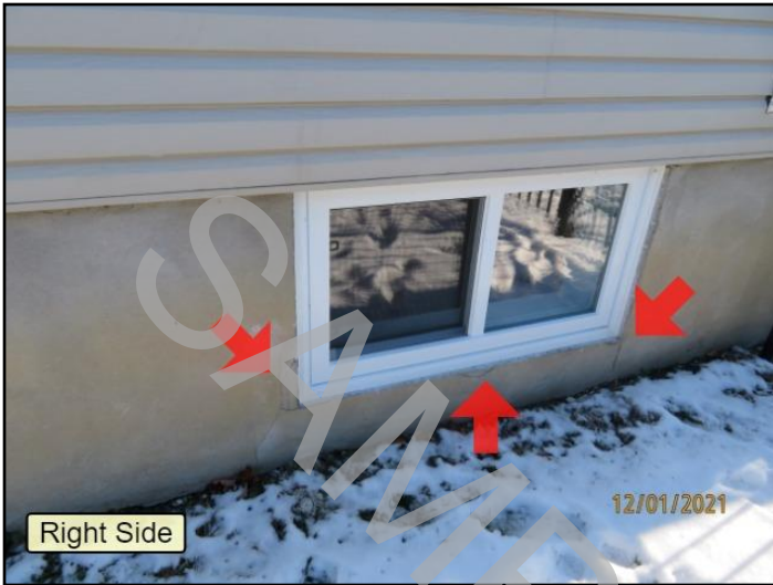
33. Grouting damaged or missing
