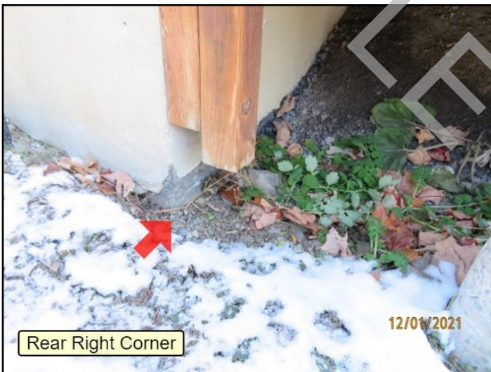
35. Grouting damaged or missing
