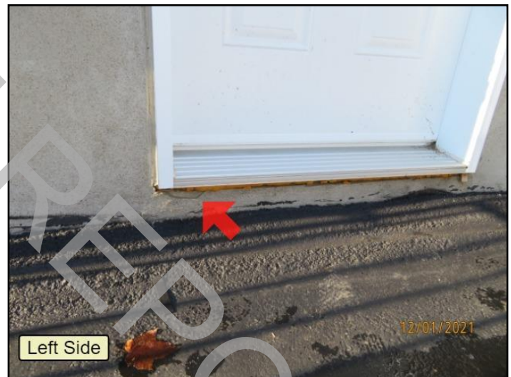
36. Grouting damaged or missing
