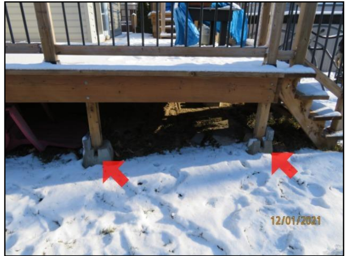
13. Poorly secured at top & bottom:At the...
