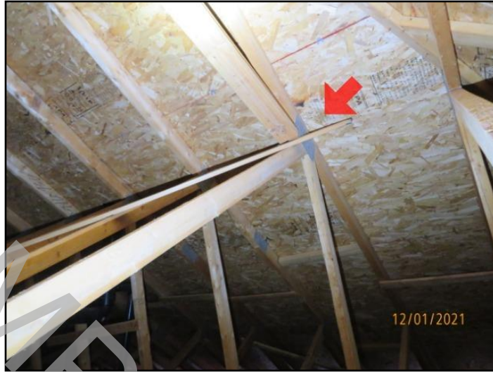
45. Poor connections
