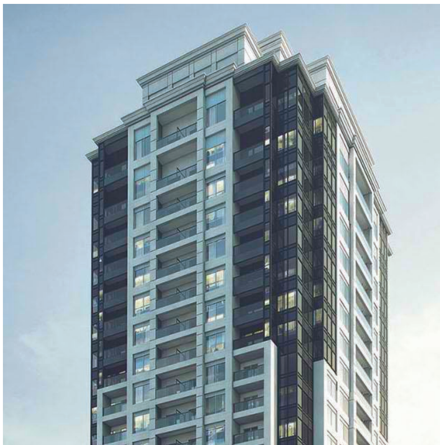
With limestone at lower levels, pre-cast and glass will characterize the upper levels, image courtesy of Devron Development
