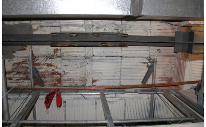
One arch retrofit using a steel T beam that provides an alternate load path
