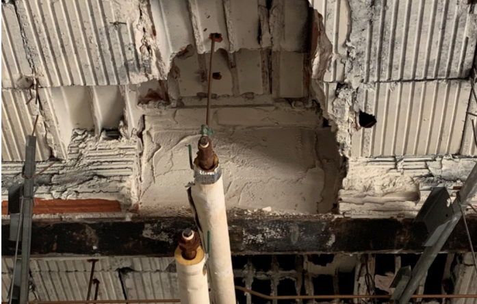
Example of damaged terracotta flat arches at Union Station Head House
