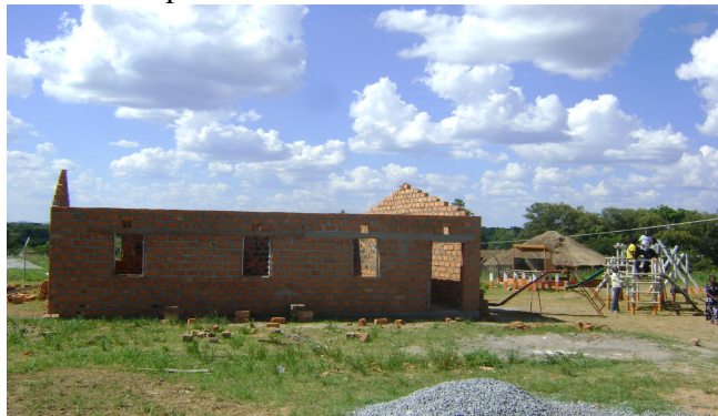
Older girls dormitory construction
