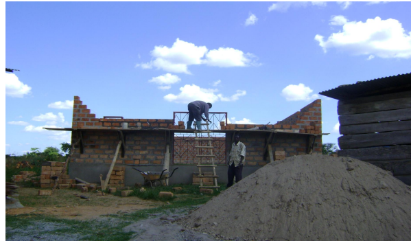
Storage room construction
