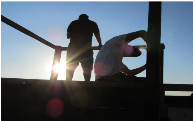
Construction of the climbing frame
