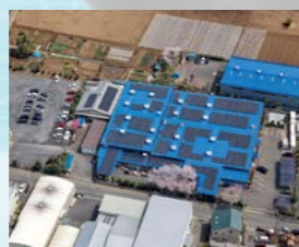
Saikama Prefecture, SHINANO INC. Head quarters
