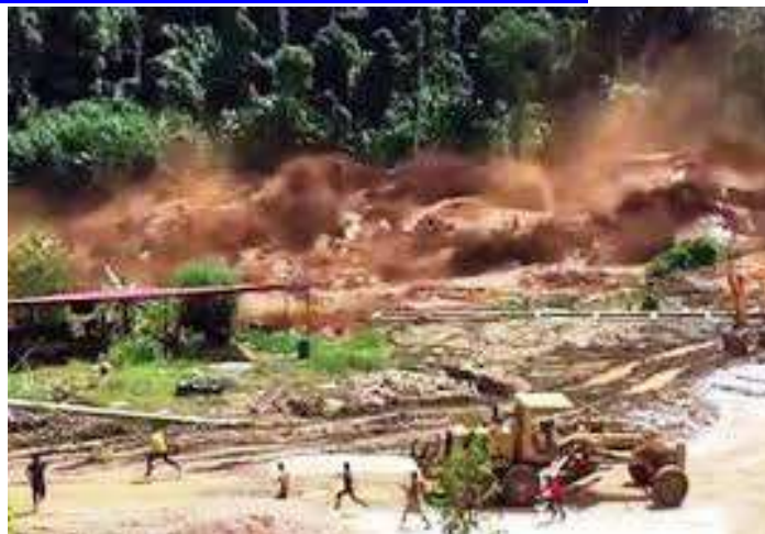
Dam breaks at Thathom district of the Xaysomboun province
