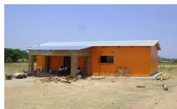
Canteen veranda now nearly finished.
