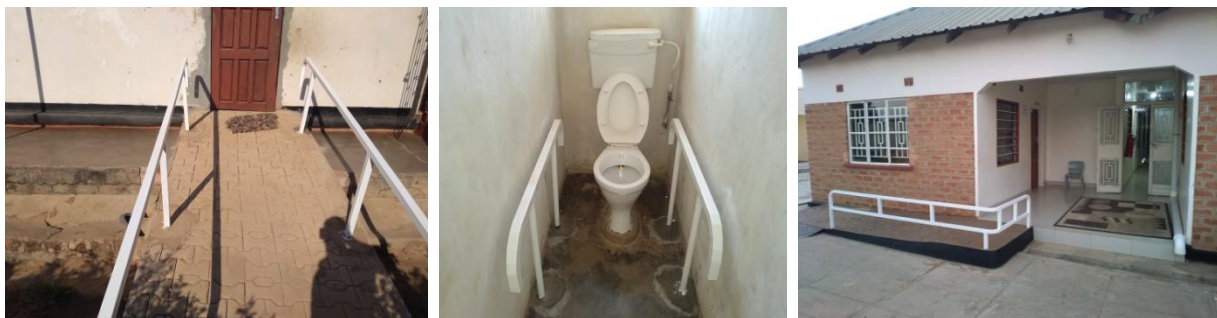
Slants for easy mobility of those using wheel chairs and those using walking sticks.
