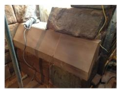
Outdoors and work carries on. It was square but now its chamfered! A block of sandstone, quarried in Cumbria and worked on by Paul, the stonemason, originally weighing about 400 cwt now sits , a little lighter, and firmly in place ,on the south wall of the Oratory.
