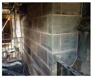
The overall effect of the repointing of the walls of the Choir and Rector's Vestry will be very pleasing, when the colour of the lime mortar mellows. Clad in scaffolding for some months, the walls will soon be bathed in sunlight once again.
