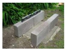
100 mm longer than the bearers also acts as a vermin guard. I then laid the two timber bearers on top of the damp proof membrane and the six thermal blocks which make up the floor of the hive were then laid flat on the timber bearers as shown in the photo below.
