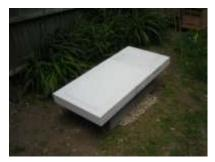
Once a level area of ground had been prepared for the slab I then compacted the soil with a an old fence post, you could of course use any other heavy object for this purpose but the more time you spend on this the less the chance of the ground subsiding unevenly under the weight of the hive. When I was satisfied with the compaction I then laid the slab on a bed of gravel some 20 mm thick and ensured that the slab was level in all directions as shown in the photo.
