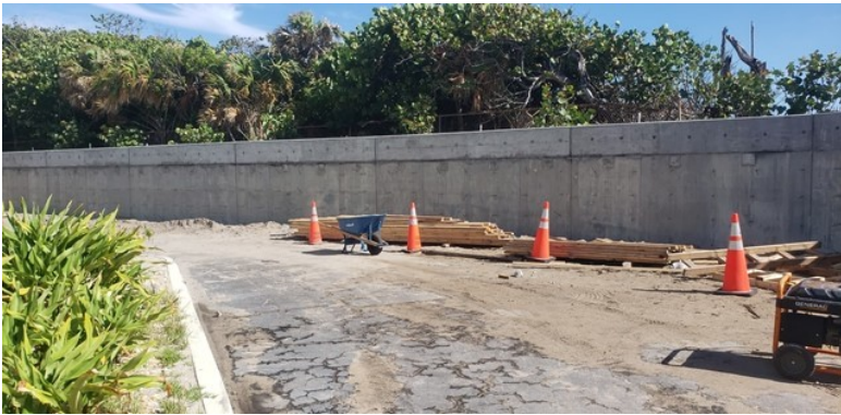
Concrete Facing to Finish Off Sea Wall Stucco & Paint to Follow
