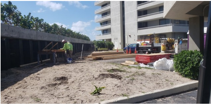
Concrete Facing to Finish Off Sea Wall Stucco & Paint to Follow
