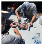
To avoid chipping on the joint edges at the moment of the installation, it is recommended to protect each joint edge with masking tape, cardboard, shims or masking tape in the border before placing the top on the base.
