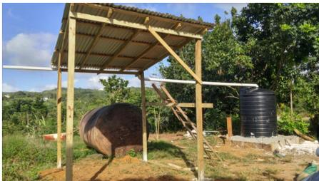
Pictured above is a completed water catchment system with water tank installed in St. Ann, Jamaica.
