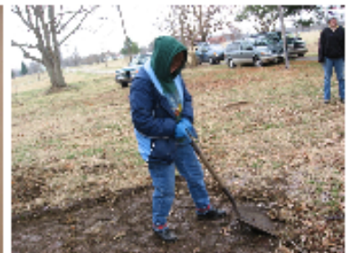
...and excavating a nice walkway
