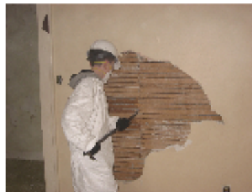
Working hard tearing out walls
