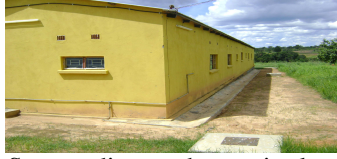
Surrounding made sure is clear
