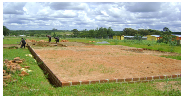
soil filling in house foundations
