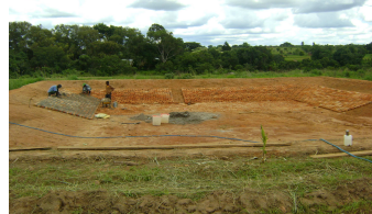
construction in progress
