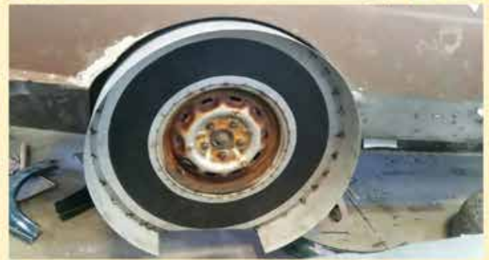
First arch now in place. Modification to the lead edge of under tank panel and rear of sill panel needed to ensure the new profile continues nicely.
