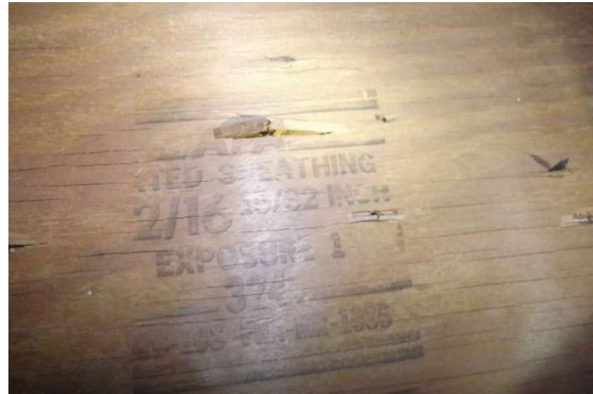
15/32" Deck Thickness Confirmed
