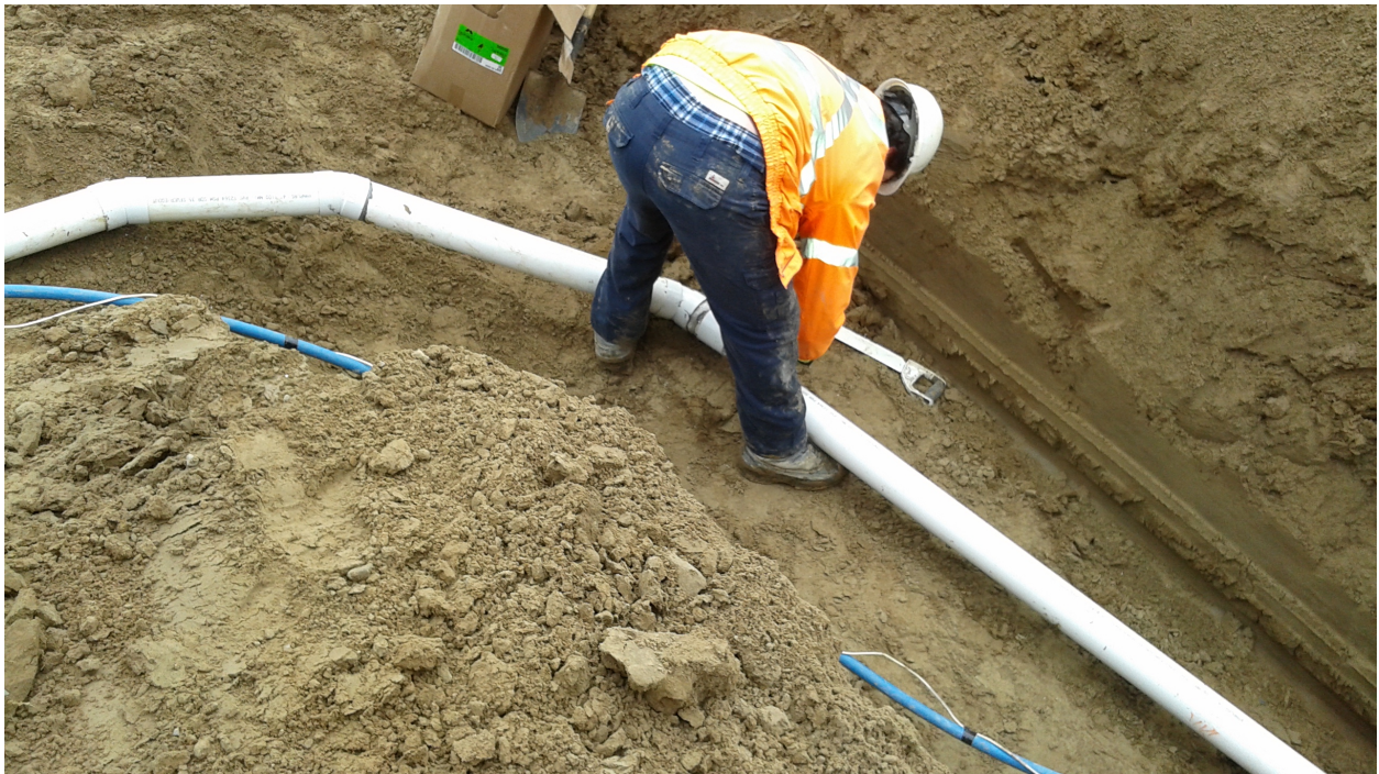
FIGURE 16: INSTALLATION OF A SANITARY BUILDING SEWER
