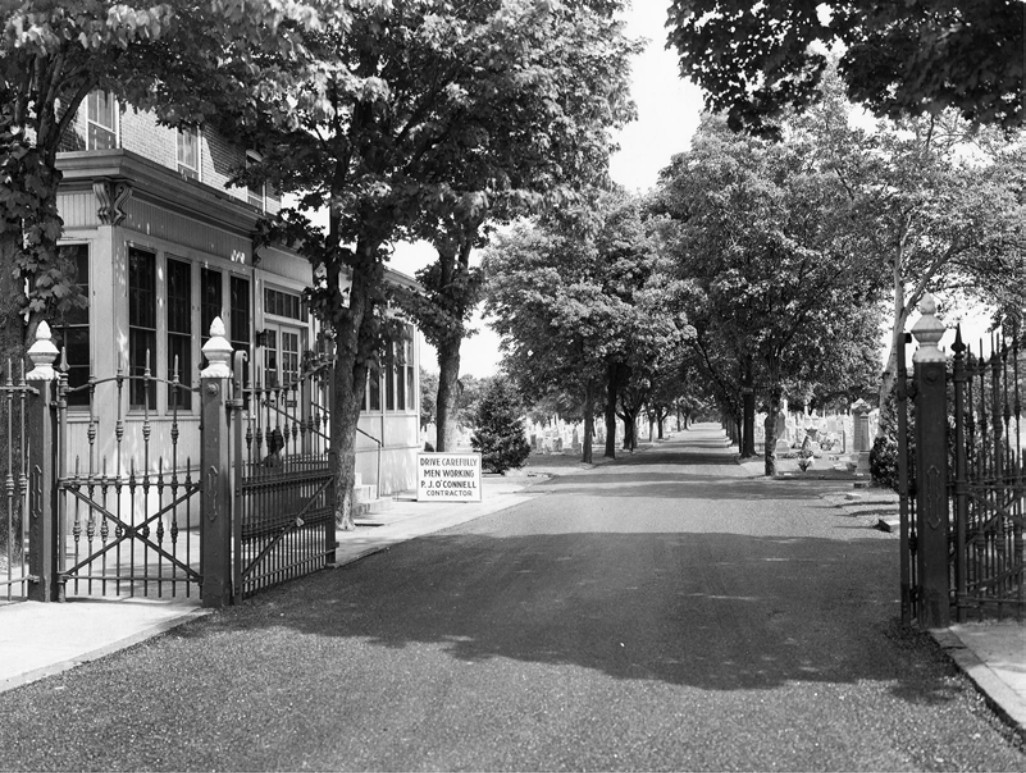
DE_New Castle County_Riverview Cemetery Superintendent's House
