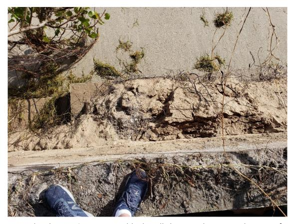
Pictured is the existing concrete block wall showing the exposed cement footer.
