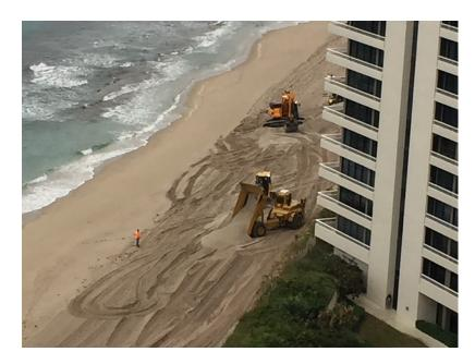
Sand was placed on dune and built up to a height of approximately the top of the overpass.
