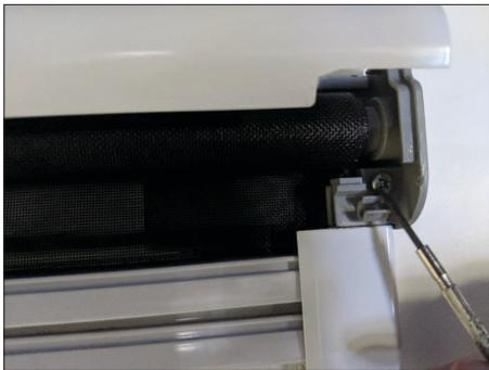
Stainless Steel lugs holding the blind assembly to the window.
