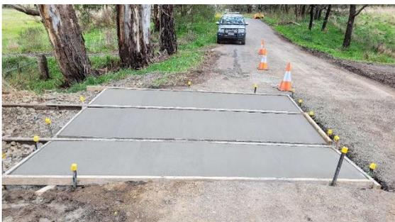
*The Tip Road is another level crossing taking shape. This road needed to be kept open, so the crossing was poured in two parts.*
