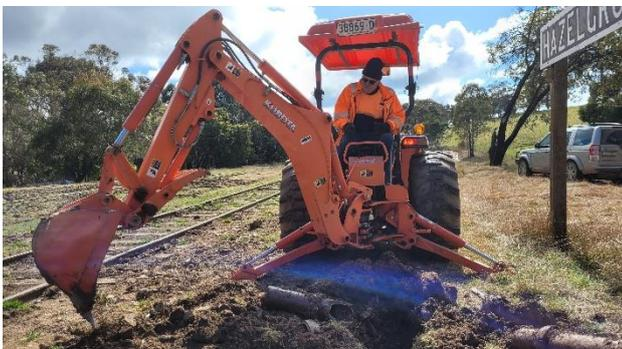
*Hazelgrove - The original ceramic pipes were blocked and had to be removed in order to get storm water away from the track*
