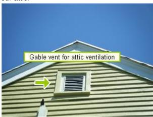
(2) Please note that one or more of the slats for the gable vent are broken -- this can allow pests to enter the attic. Recommend having a contractor or handyman repair the slats and install a screen behind the gable vent to help keep pests out.
