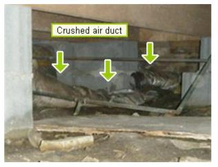
(2) As viewed from inside the attic, observed that one or more of the air ducts are sagging. For your reference, air ducts that aren't well supported can leak, condensation can form and drip onto the ground and/or air flow may be reduced which means that areas in the house may not be as comfortable as they could be. Recommend having a contractor or HVAC repairman add support for the ducts so they hang as straight as possible to facilitate good air flow.
