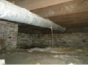
(2) As viewed from inside the crawlspace, observed that part of the main floor beam (which runs from the front of the home to the rear) is damaged in one section located near the front
