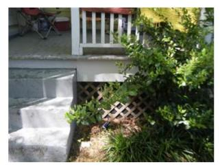
(2) Observed that some of the lattice screen which encloses the crawlspace has been opened -- this will allow pests to enter. Recommend having a handyman replace the sections of lattice screen which are damaged and install a screen behind them to help keep pests out.
