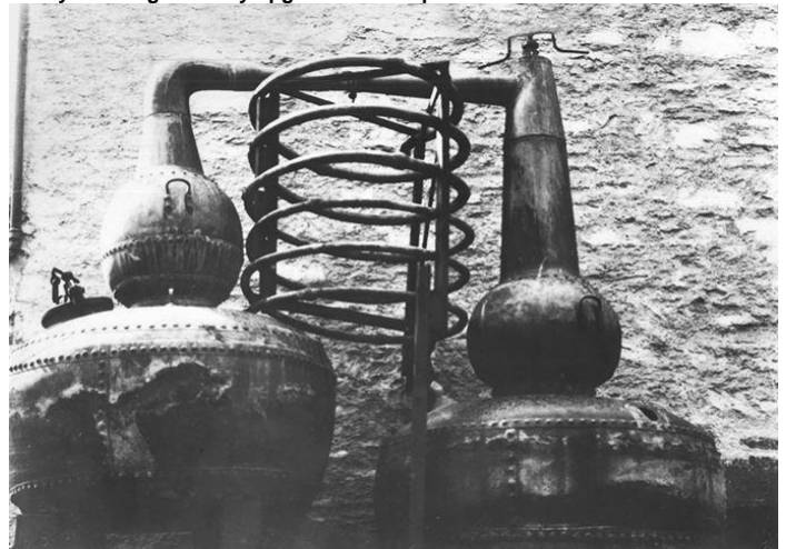
'Old-fashioned' setup: Stromness distillery's two 'sma' pot stills, 1913 (Photo: Orkney Library and Archive)
