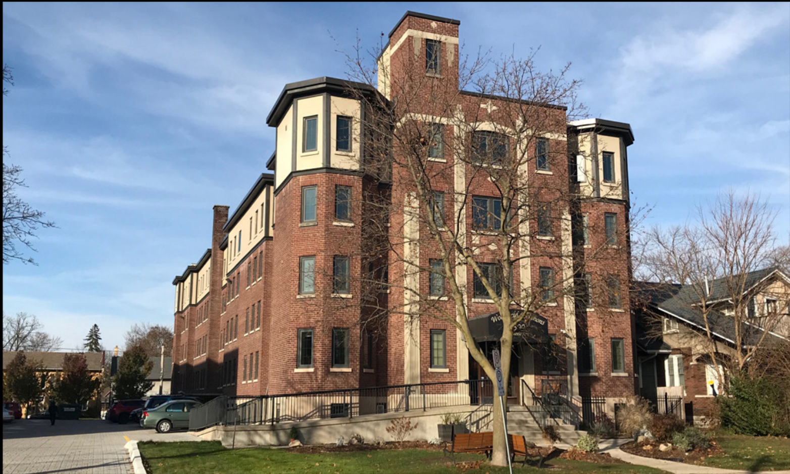
The Jarvis building - now 'Woodfield Commons' (a geared-to-income housing conversion in West Woodfield)
