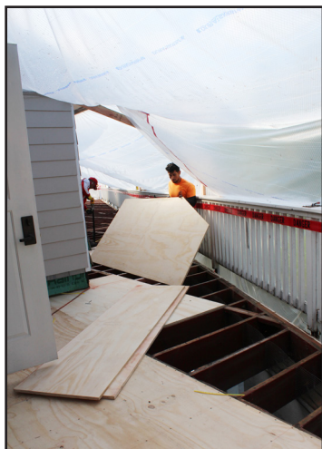
Construction worker laying the plywood for the new deck on Building C
