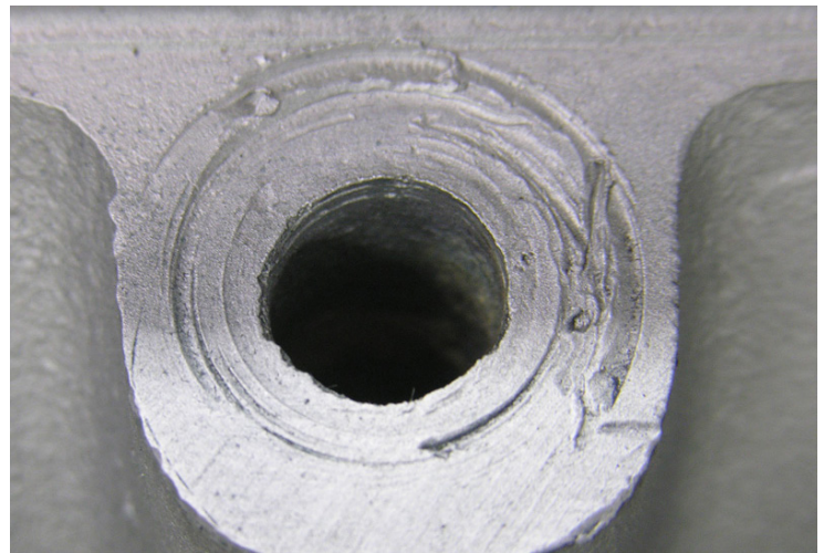
Another area that can require attention is gouging of the washer surface from the acorn nuts that hold the cylinder head down. This gouging is caused by someone in the past tightening the head down without flat washers installed.
