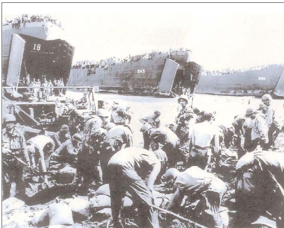
D-Day at Leyte. Soldiers fill sand bags to create sand road to ramp of LST-18.
