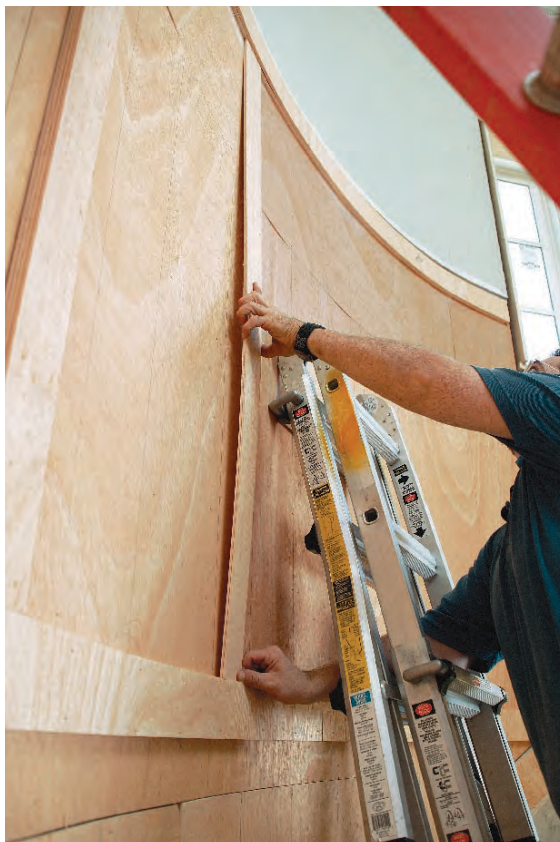
A second doubled layer of bending lauan forms the rails and stiles.
