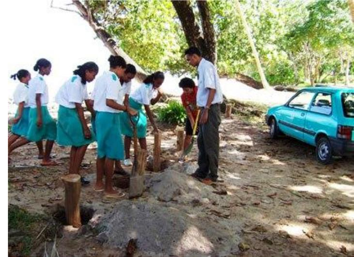
*•As means of coastal protection the Environment Department has in the past installed wooden pickets, but the effort was not a success as they were not concretized. Concrete bollards have been installed at North East Point and have proved to be very effective and difficult to remove. Rock armoring was also implemented in some areas.*
