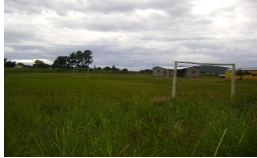
Football pitch repaired
