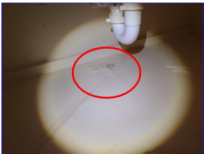
A. Item 4(Picture) Evidence of previous leak under the lavatory in the upstairs hallway bathroom. Recommend monitoring for leaks in this area.
