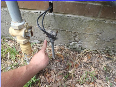
A. Item 1(Picture) Loose clamp on grounding rod/wire under the gas meter at the right side of home.
