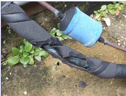
B. Item 4(Picture) Recommend repairing damaged insulation on a/c suction line at the condenser on the right.
