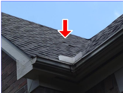
C. Item 1(Picture) Nail pops noted at front facet of home above the front entrance.
