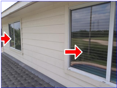
H. Item 2(Picture) Missing screens on windows at back of home.
