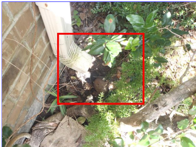
B. Item 1(Picture) Missing splash block/downspout extension at back right corner of home. Recommend installing to help prevent erosion and damage to property
