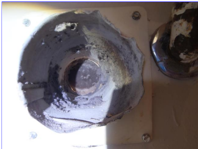
H. Item 1(Picture) Slight bit of debris in the dryer exhaust.
