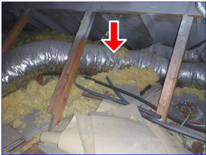
C. Item 2(Picture) Duct laying in insulation at time of inspection.
