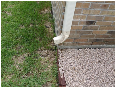
B. Item 3(Picture) Missing splash block/downspout extension at back left corner of garage.
