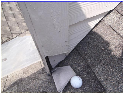
J. Item 1(Picture) Damaged trim on exterior of chimney.
