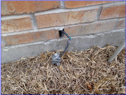
A. Item 2(Picture) Loose clamp on grounding rod at meterbase.
