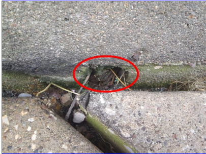
A. Item 2(Picture) Exposed post tension end at the left side of home near the back by the driveway.
