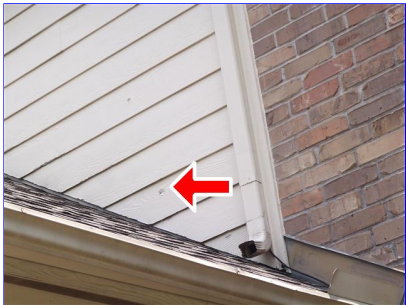
E. Item 4(Picture) Slightly damaged siding at the front left side of home.
