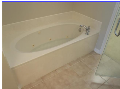
D. Item 1(Picture) Missing access panel for hydro massage tub. This may not have been required when the home was built but should be installed to be able to inspect plumbing.
