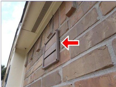
E. Item 3(Picture) Recommend sealing around vent on exterior wall at the left side of home to help prevent moisture intrusion.
