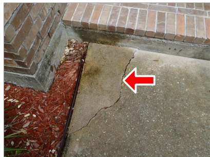
L. Item 1(Picture) Damaged flatwork at the front of home by the front door.
