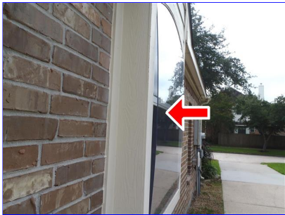
H. Item 1(Picture) Loose piece of excess glass on exterior of window at the left side of home. Unsure of purpose of this but recommend further evaluation and repair as needed.
