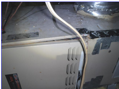
A. Item 5(Picture) Loose cover on furnace number two at time of inspection.
