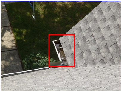
B. Item 6(Picture) Ponding water in gutters at front of home above the front entrance.
