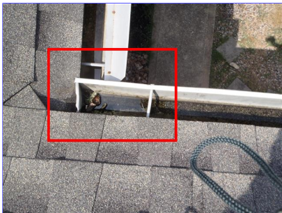
B. Item 5(Picture) Ponding water in gutters at back of home at time of inspection.
