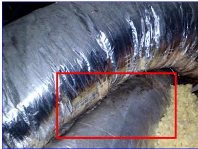
C. Item 1(Picture) Touching and condensating ducts noted in the attic at the by furnace number two.
