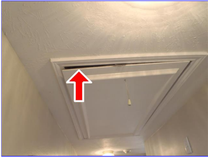
D. Item 1(Picture) Gap in upstairs attic hatch.
