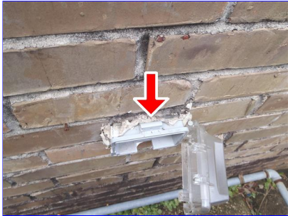
E. Item 1(Picture) Recommend re-sealing around electrical, by the a/c condensers at the right side of home, to help prevent moisture intrusion.
