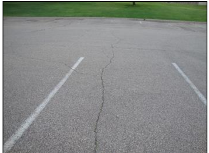
Major repairs to the asphalt pavement...
