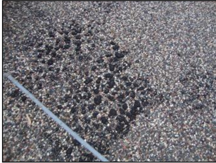
Blistering, which occurs when air or...
