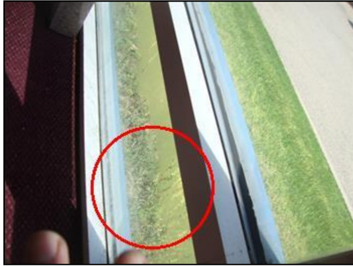
A lost seal has resulted in the formation...
