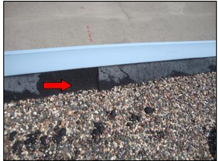
The membrane is exposed to sunlight damage...
