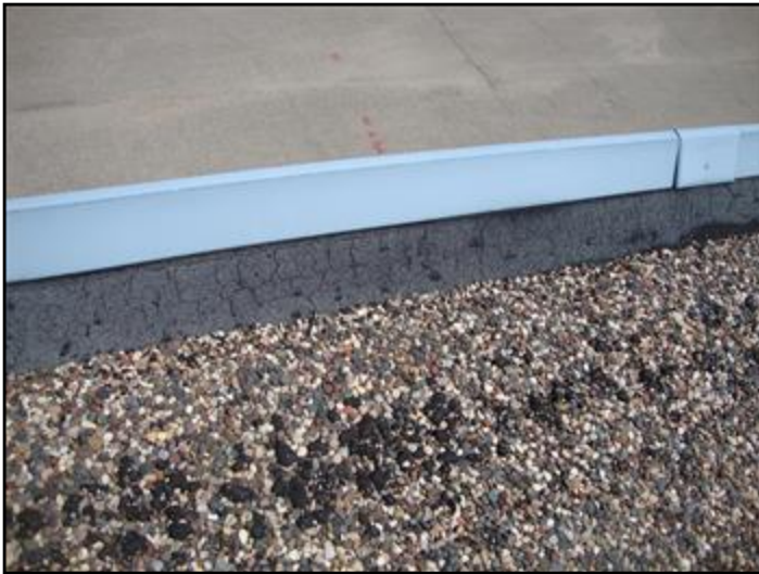
The membrane is exposed to sunlight damage...
