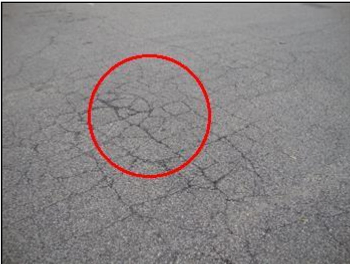
Major repairs to the asphalt pavement...
