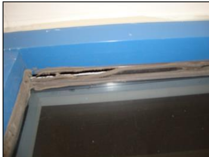
Deteriorated caulking
