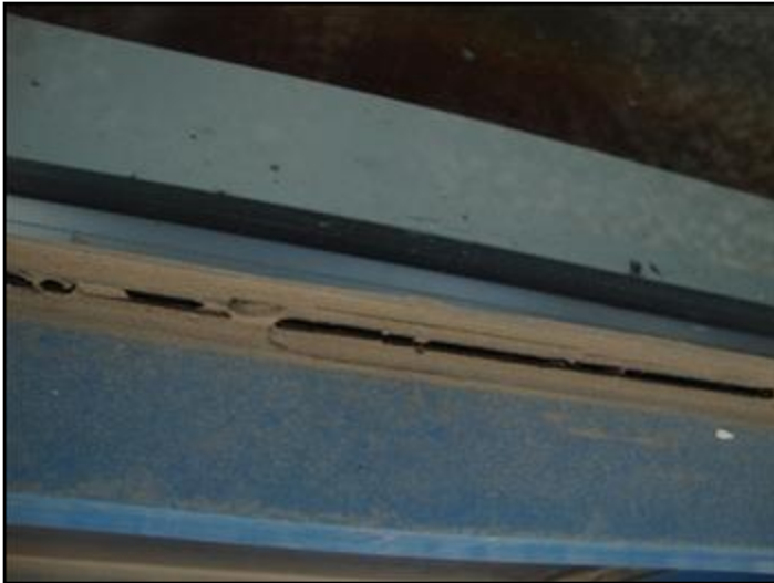
Deteriorated caulking
