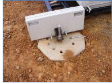
Frame Fastened to Concrete Pedestal at each Corner
