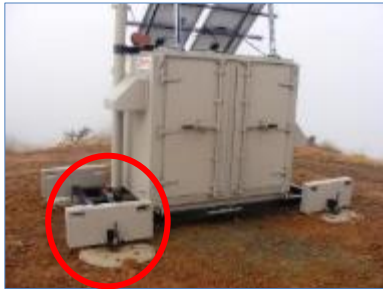
Ballast Plates Installed on Each Corner of the Frame
