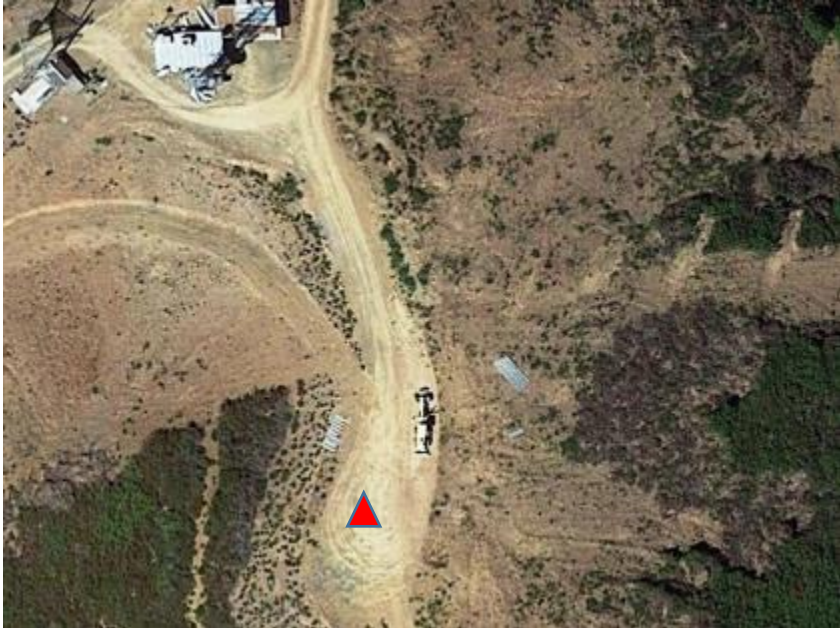
Top View of Facility
