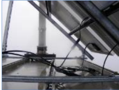
Solar Panel Support Frame Fastened to Top of Cabinet
