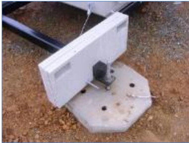
Steel Ballast Plates Installed at Each Corner
