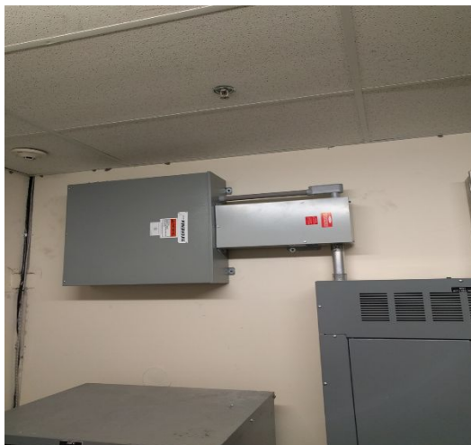
480 Volt / 100 KVAR Powerhouse can be installed in various positions as shown above
