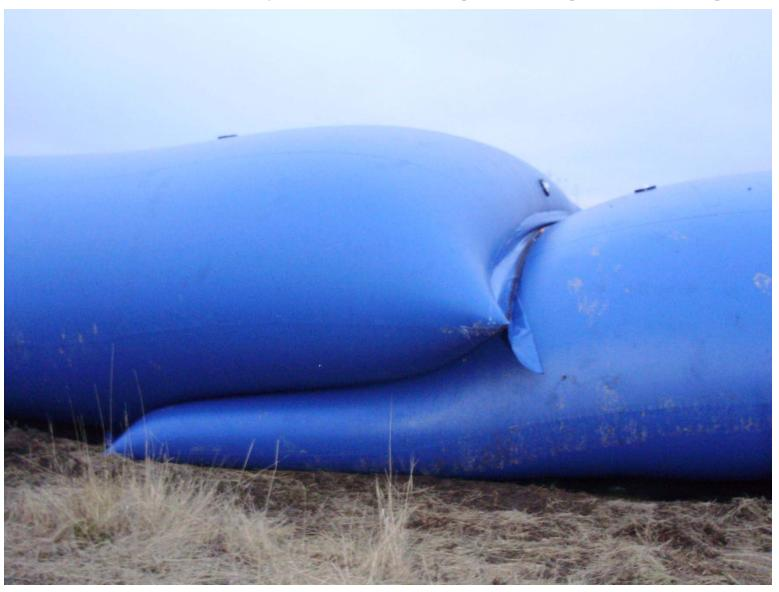
When inflating on an incline measure the height of the WIPP at the lowest point of gravity to ensure WIPP is not overinflated
