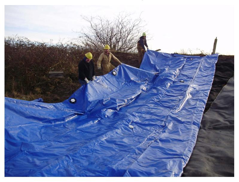
With the first WIPP in place position next WIPP on top and unroll into position using the correct amount of overlap. 8ft high WIPP requires 12ft of overlap.
