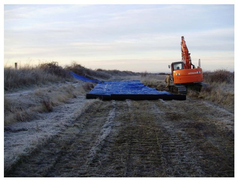
Install a sheet of geo textile first then install WIPP on top of the protective membrane to protect WIPP from damage
