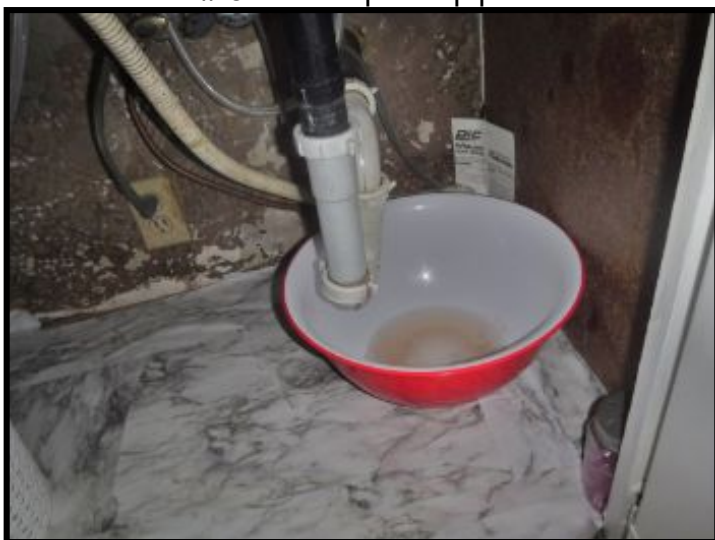
#19. Leaking under sink.
