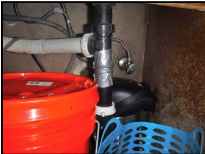
# 5. Duct tape on pipe.
