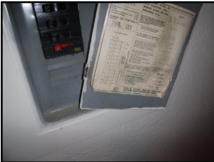
#10. Panel door needs to be secured.
