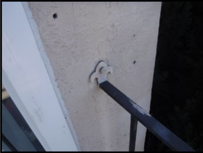
#10. Railing needs securing.
