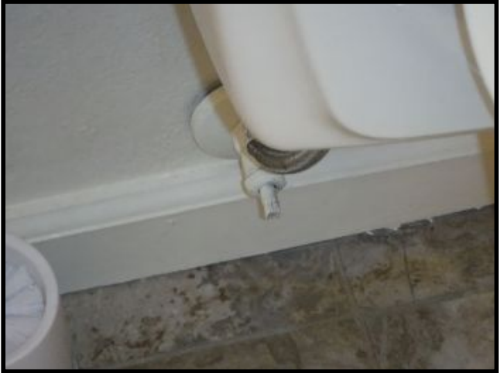
#30. Shut off handle missing.
