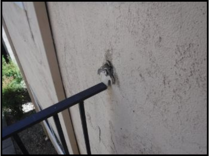
#31. Railing not secure.
