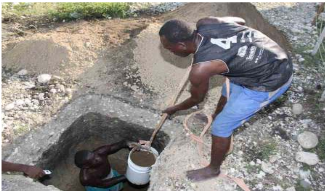
Fig. 2. Improper and unsanitary toilet systems where bayakous are used (Fortuné)
