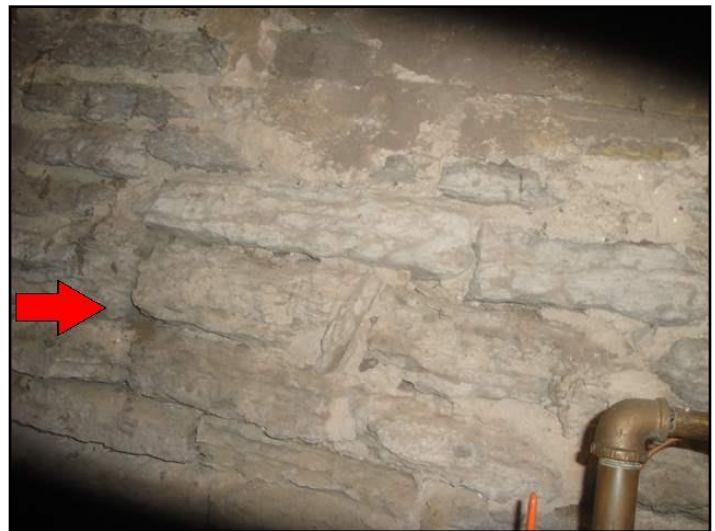
38. Spalling, crumbling or broken material
