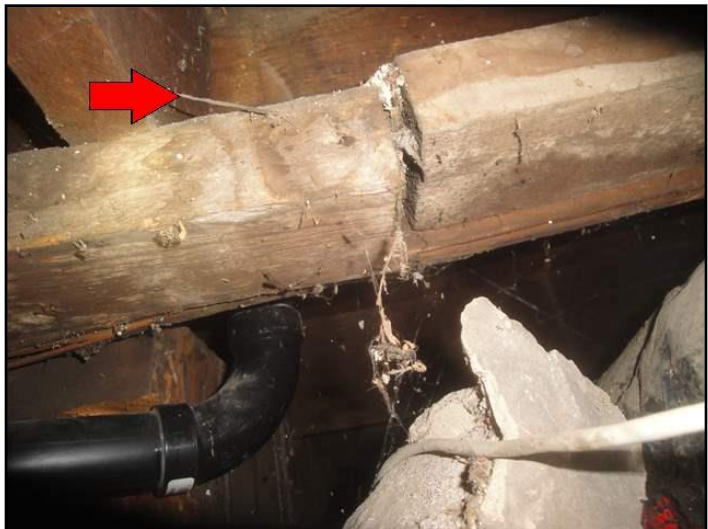
48. Poor end bearing, joist hanger connections
