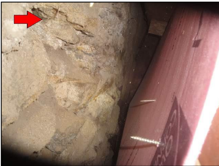
37. Spalling, crumbling or broken material
