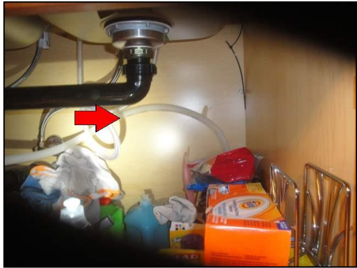
76. Dishwasher drain connections
