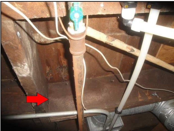
47. Poor end bearing, joist hanger connections
