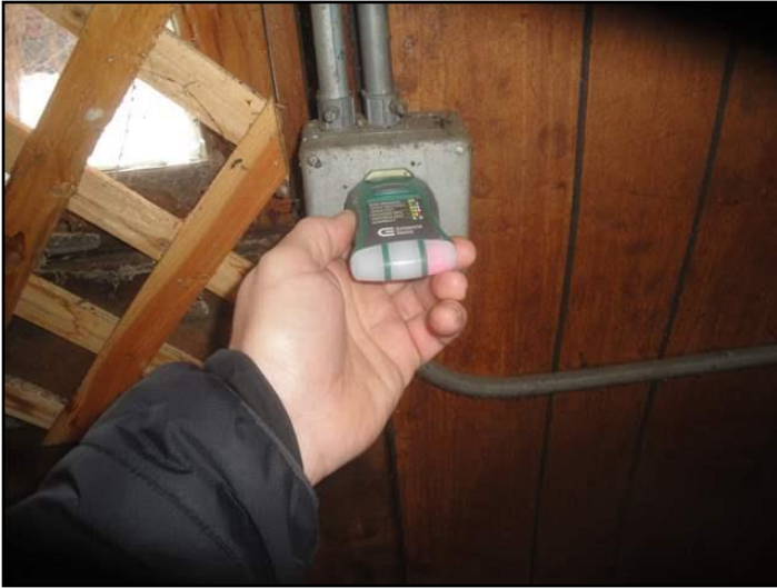
66. Ground needed for 3-slot outlet
