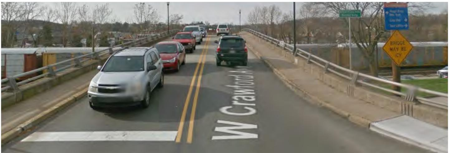
*Safety problems currently represent barriers to bicycle and pedestrian mobility within Connellsville. The Crawford Bridge crossing shown here is one example, combining heavy vehicle volume, slope, narrow sidewalks and low safety railings.*
