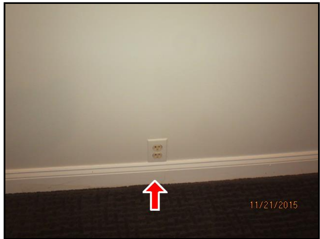
3.3 Item 2(Picture) Low outlet
