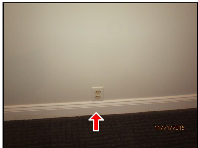
3.3 Item 2(Picture) Low outlet
