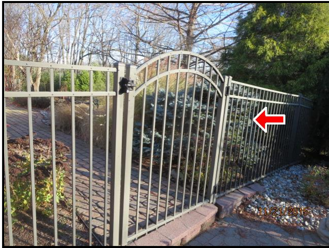
11.15 Item 1(Picture) Gate
