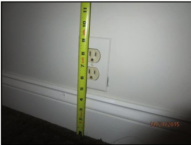
3.3 Item 1(Picture) Low outlet
