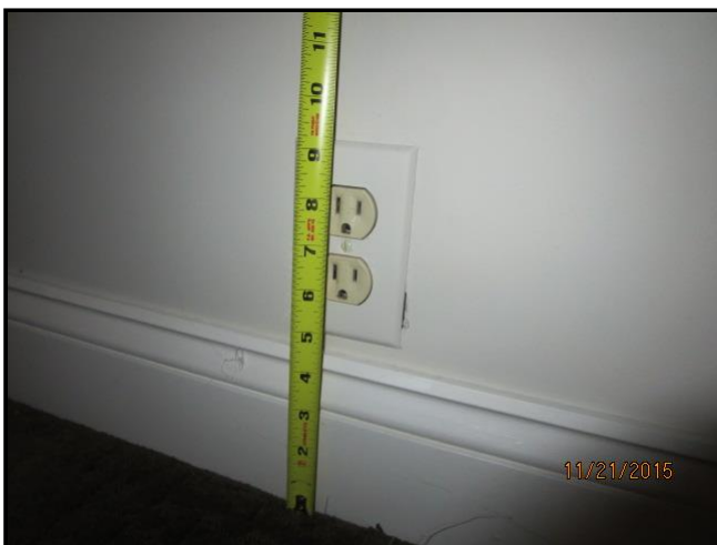
3.3 Item 1(Picture) Low outlet
