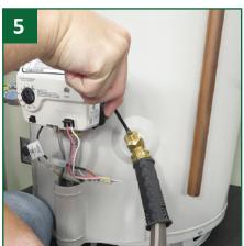
Drain and flush tank (very important for gas water heaters). Turn off cold water supply, and open drain valve. Open T&P relief valve to relieve pressure. Drain 2-3 gallons of water. If water is milky, drain entire tank. Close drain valve and open cold water supply valve. Open a hot water faucet and let hot water run 3 minutes to make sure all air out of tank before returning to service (very important for electric water heaters).
