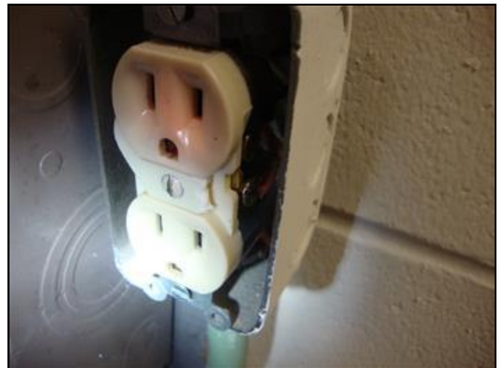
7. Missing on switches, outlets and junction...
