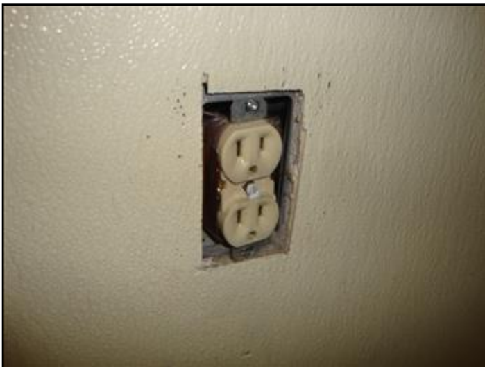
6. Missing on switches, outlets and junction...
