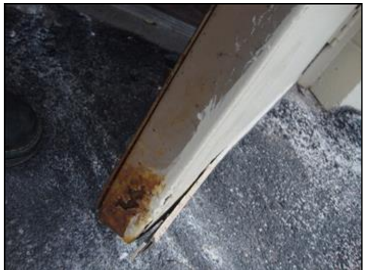
53. Corroded
