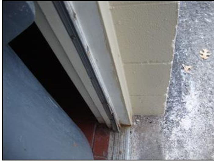
54. Corroded
