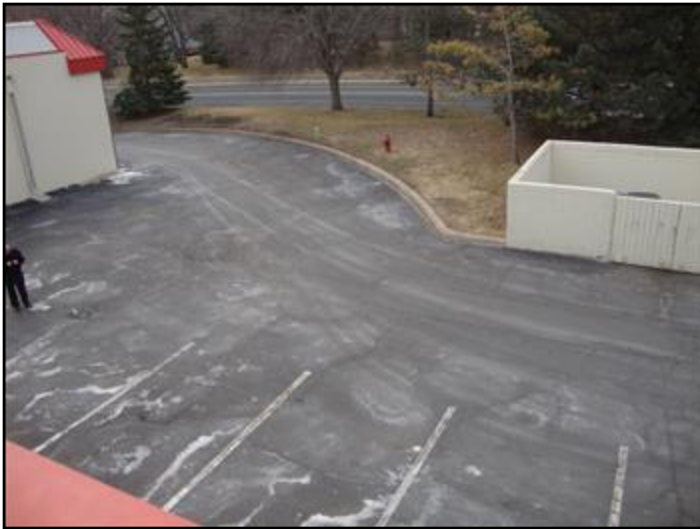
60. Poor overall condition
