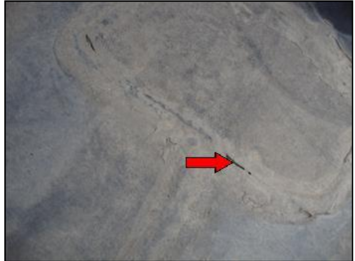
19. Open seams at lap joints
