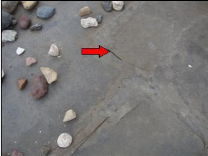
18. Open seams at lap joints
