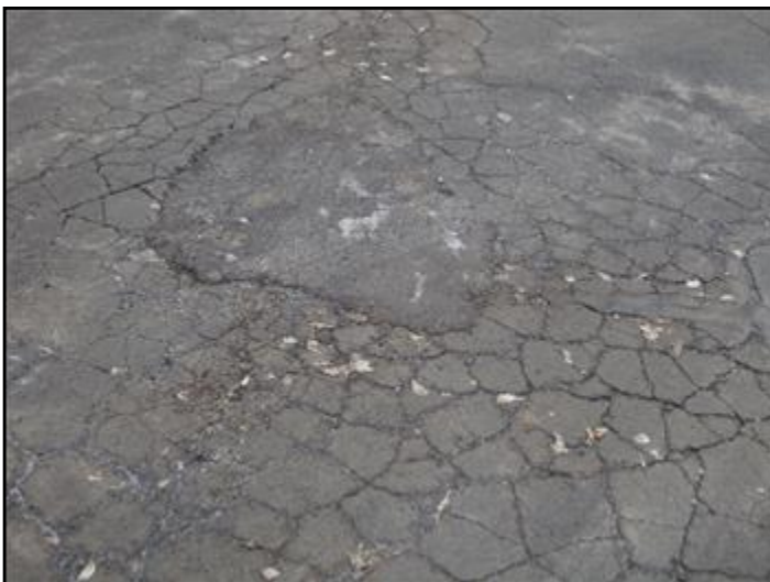
62. Poor overall condition
