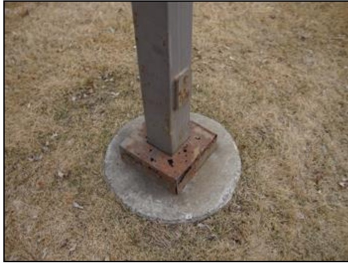
64. Corroded lighting
