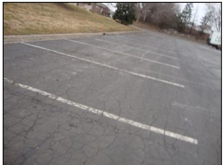
63. Poor overall condition
