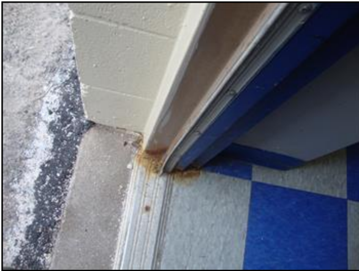
50. Corroded
