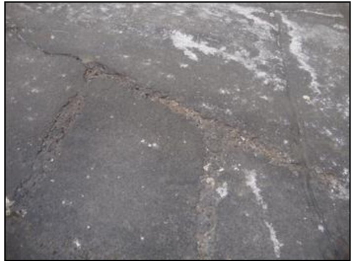
61. Poor overall condition
