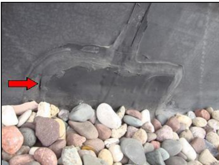
20. Open seams at lap joints
