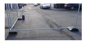
In all cases more ballast may be used and in the interest of safety to all use ballast posts connected to main fence using two clips
