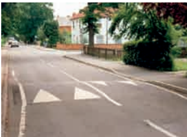
Fig. 4.5 Round-top (left) and flat-top humps
