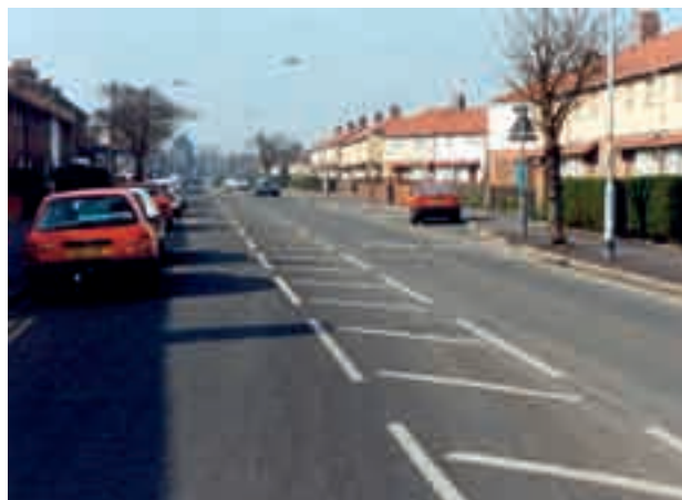
Fig. 10.2 Hatched road markings
