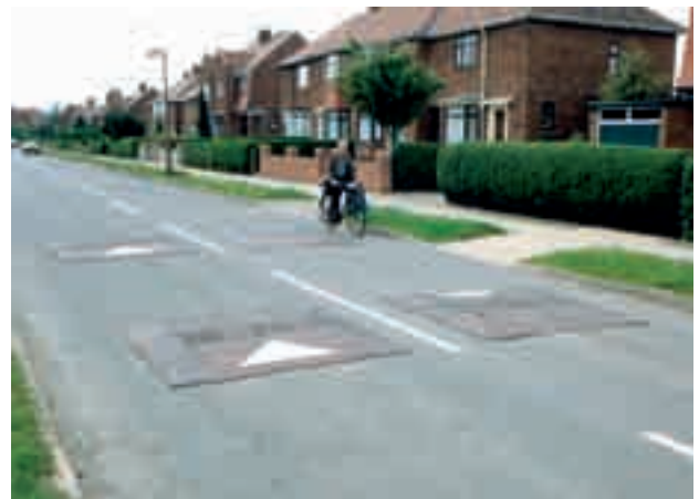
Fig 4.15 Speed cushions (left to right: two abreast, three abreast and double pair)
