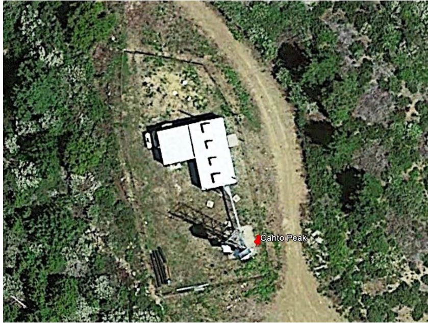
Top View of Facility
