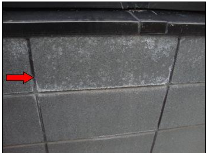
Efflorescence
