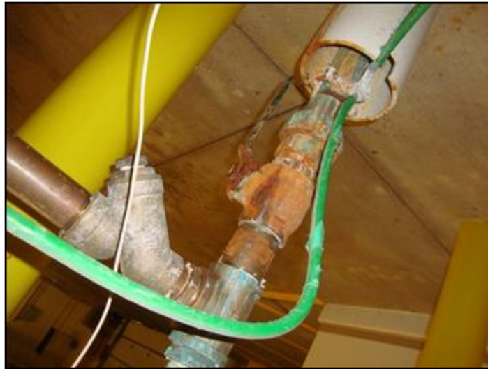
Corrosion
