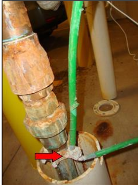
Corrosion
