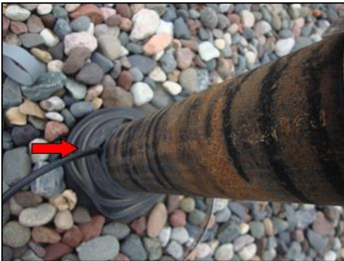
Wire in boot flashing
