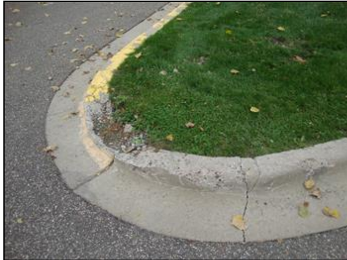
Curbing damaged
