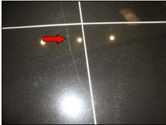
Minor cracks
