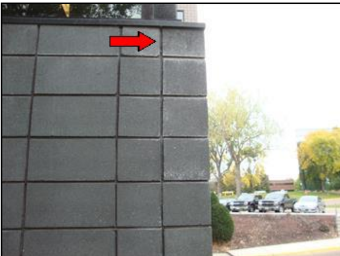
Efflorescence
