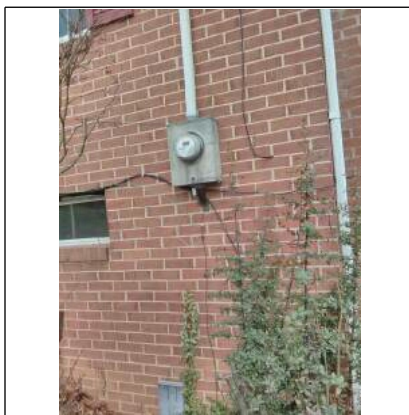
Electric meter/meter box
