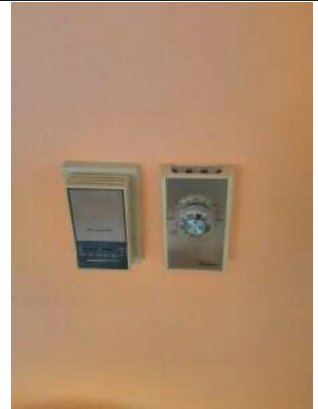
AC thermostat left heat thermostat right
