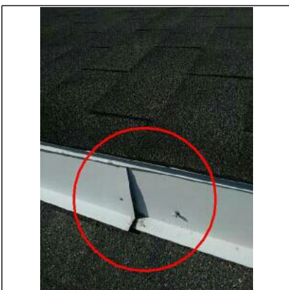
Loose Flashing
